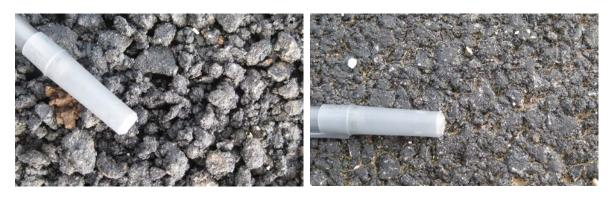
Figure 2 – Segregated asphalt can lead to coarse texture (a) within a meter of fine texture (b)
