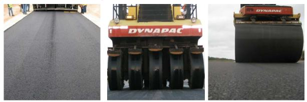
Figure 6 – Streaking from poor paving practice (a) and pneumatic (b) and steel drum (c) compaction
