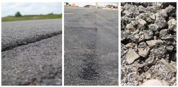
Figure 1 – Poor joint construction (a,b) and deteriorated asphalt material (c)
