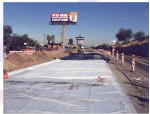
Figure 1. Pavement protected with polyethylene sheets.
