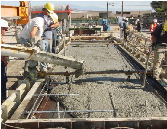
Placing concrete in forms for the California project.
