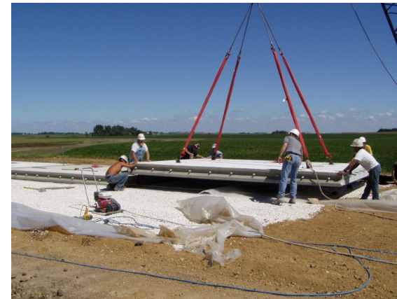
Installation of a panel for the Iowa bridge approach slab project.
